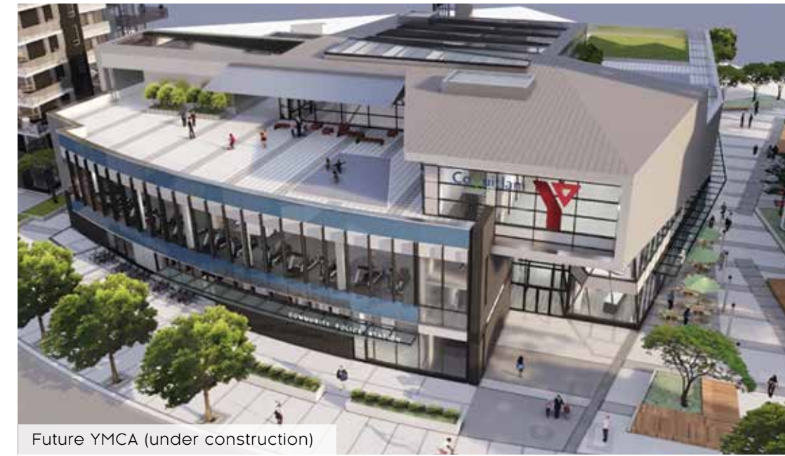
Future YMCA (under construction)
